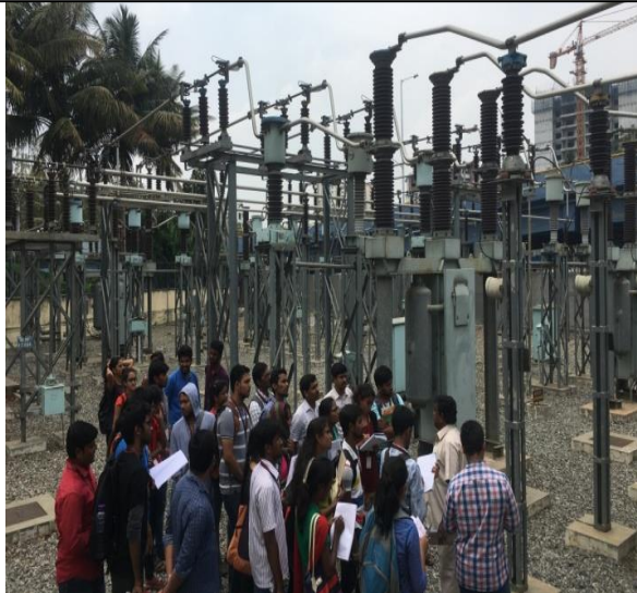
Our Students at 400/220KV Substation
