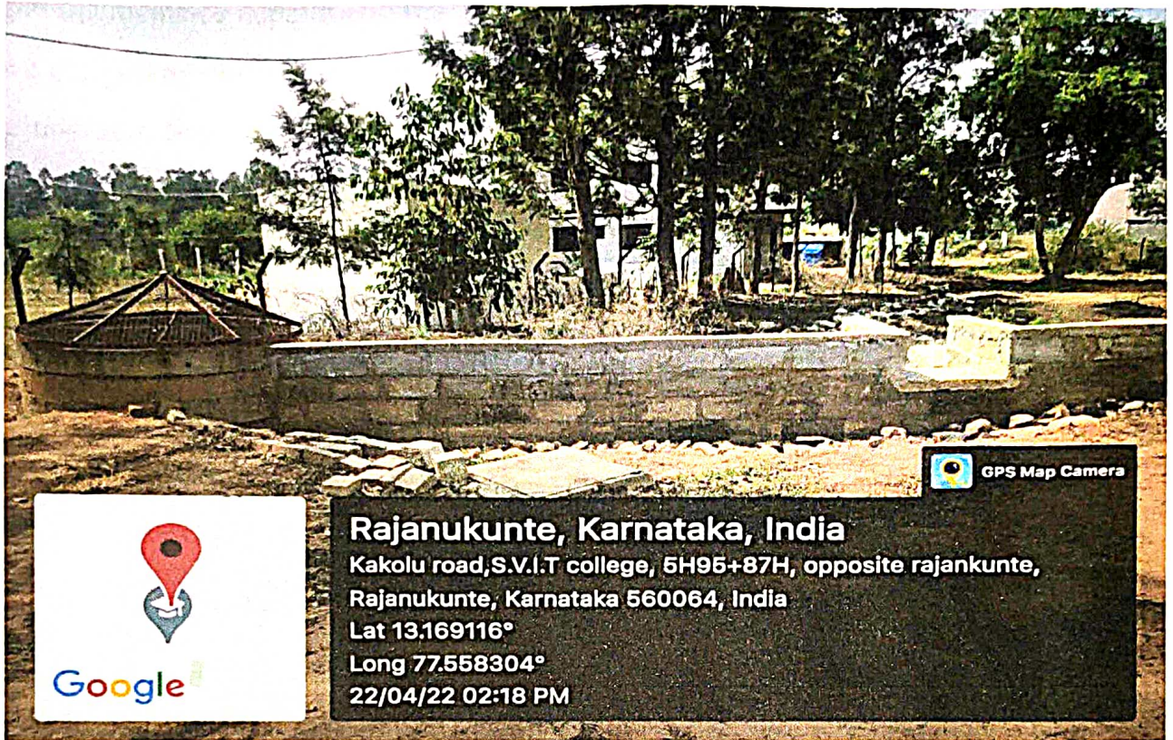
Check Bund with recharge well
