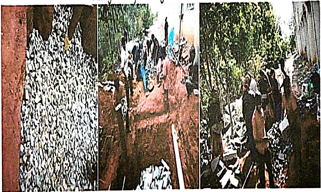
Filling second layer of 40mm aggregates jalli stones
