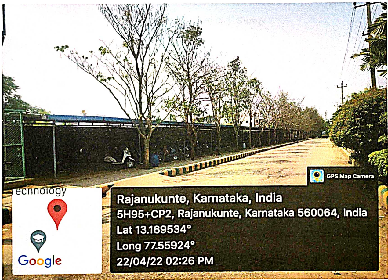
Roof top rain water collection from parking lot
