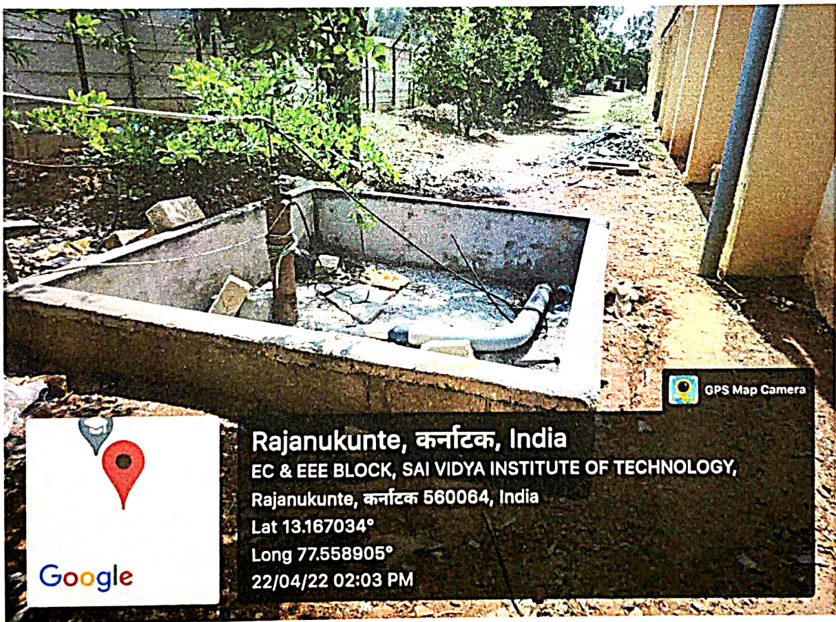
Recharging of Bore well by roof top rain water and from land discharge
