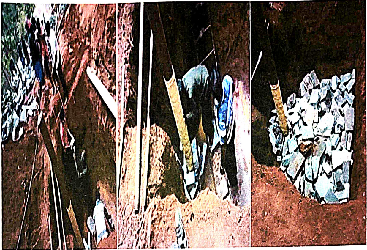
Filling first layer of big sized boulders stone
