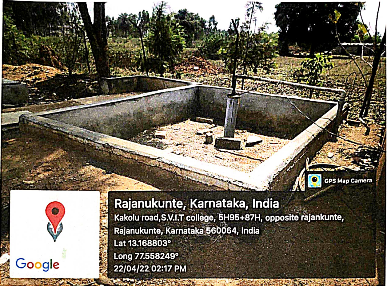
Recharging of Bore well by roof top rain water from Block 3 & from land discharge
